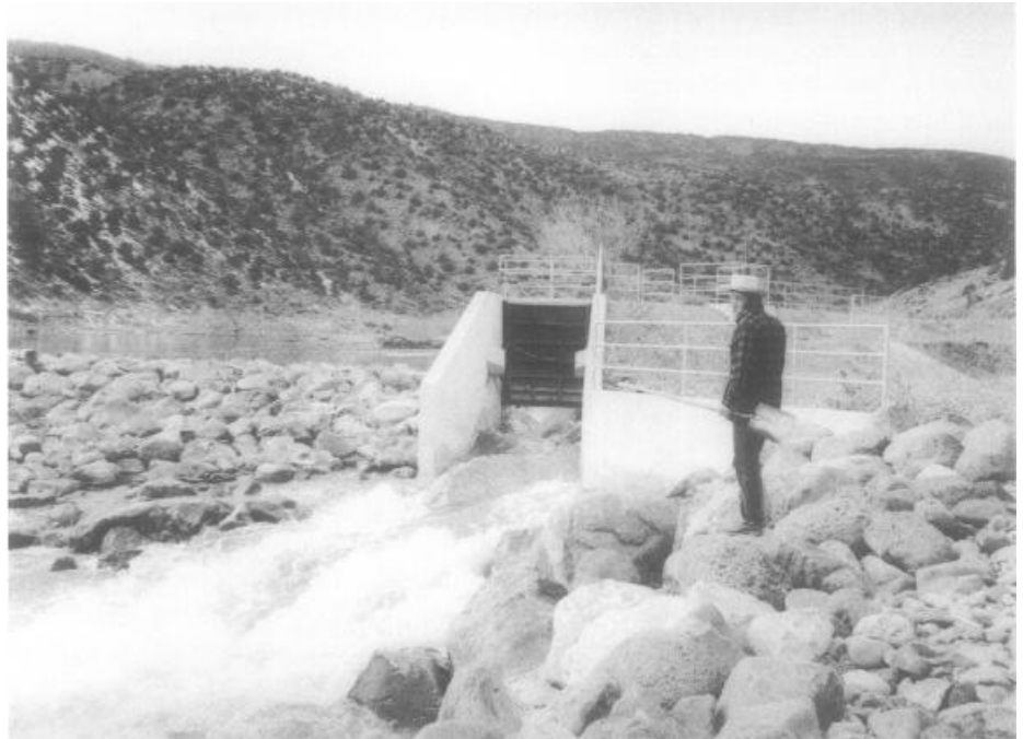
In Velarde, N.M., a new diversion dam on the Rio Grande is improving water flow into community-controlled irrigation ditches, or acequias. Foundation support aims to help the rural poor make the best use of land and water resources.
