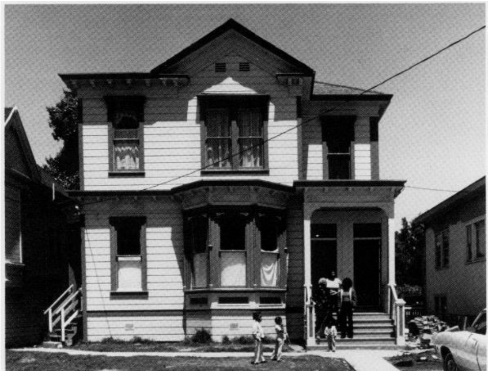
This old house in Oakland, California, shown before and after rehabilitation, was converted into apartments for low-income families. Financing was arranged by a community organization with the assistance of the Local Initiatives Support Corporation.
