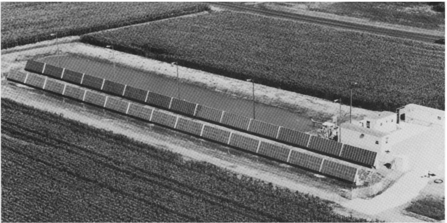
The Foundation this year provided funding for studies of decentralized generation of electric power and solar-based facilities. At Washington University a group is examining new energy systems on farms, such as this solar collector in Nebraska which is converting the sun's energy into electric power to pump water for an irrigation project.
