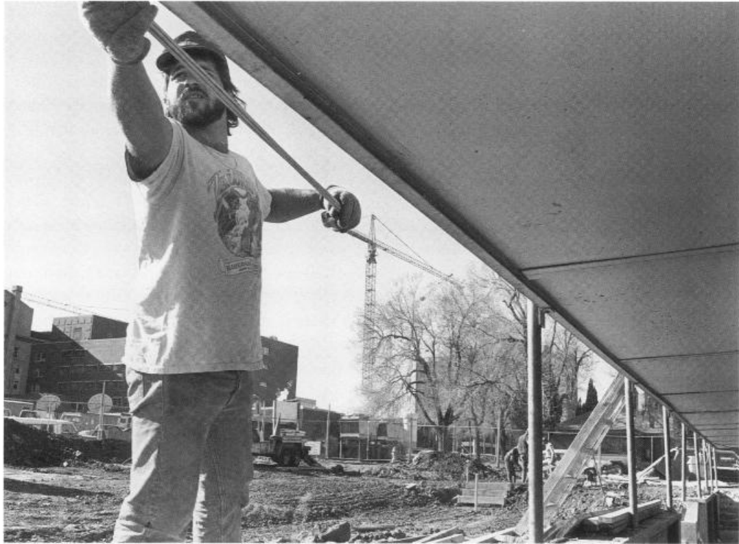
Workers completing Uptown Gardens, a low-income housing project of a Denver community development corporation (CDC). Support for the CDC movement has been a cornerstone of the Foundation's efforts to revitalize distressed urban communities.
