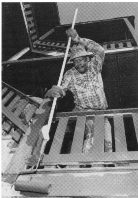
The Enterprise Foundation has received both loan and grant support to improve housing in poor neighborhoods. Here, a resident of a Chicago project contributes "sweat equity" to satisfy part of his down payment.
