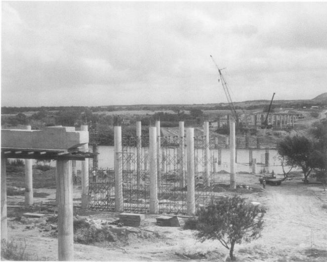
A new bridge from Mexico over the Rio Grande is being built to prepare for an expected jump in trade with the United States—the subject of a $200,000 study grant to the Autonomous Technical Institute of Mexico.
