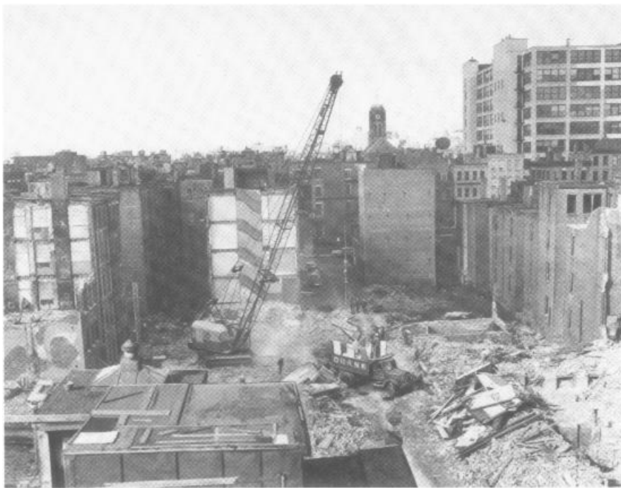
Demolition of twenty acres of south Boston slums is initial step in urban redevelopment program now under way following metropolitan area research
